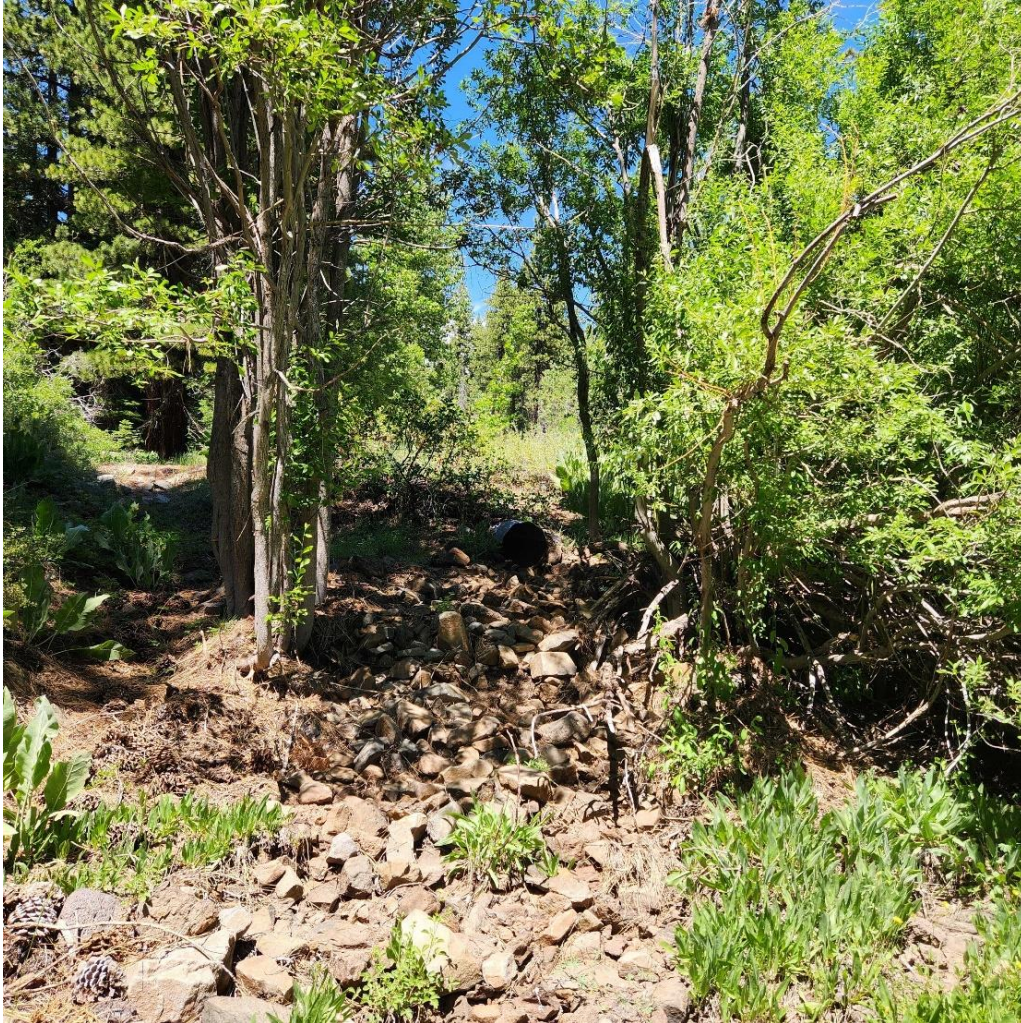
Photo 4. South side of trench alignment at road culvert.
